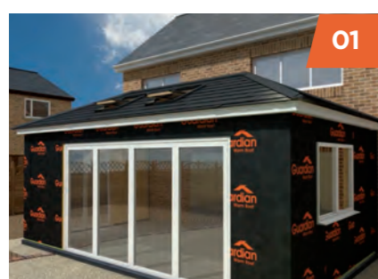
01 Breathable waterproof membrane is secured to the Kingspan TEK® walls.
