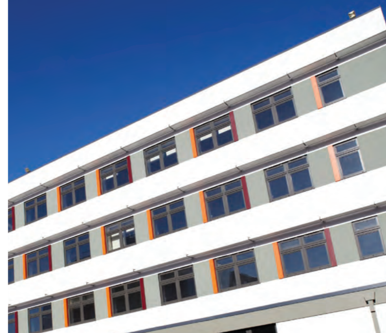
Lowery Centre - Waltham Forest College
