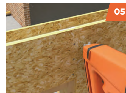
05 Wall panels are securely fixed together with a nail gun.
